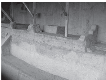
IMS adventurers got to see first hand the various constructions methods visible in the in the site's main archaeological excavation area. Note the pedrin visible behind the outer plaster. Photos courtesy of George And Audrey DeLange. They've got great coverage of many Maya sites at: http://www.delange.org .
