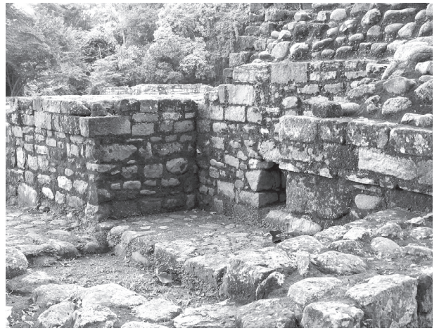
Copán masonry of tuffa ashlar bedded in clay mortar.
