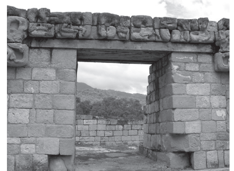
Copán Temple 22 showing Petén-style wood fixed-end lintel embedded in the masonry.
