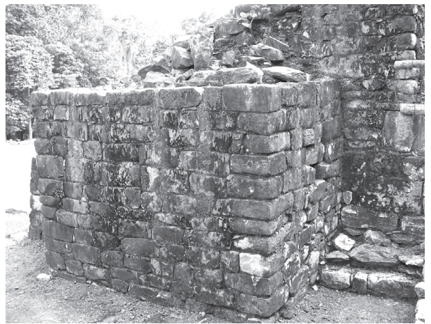
Quiriguá masonry of tuffa ashlar bedded in clay mortar.
