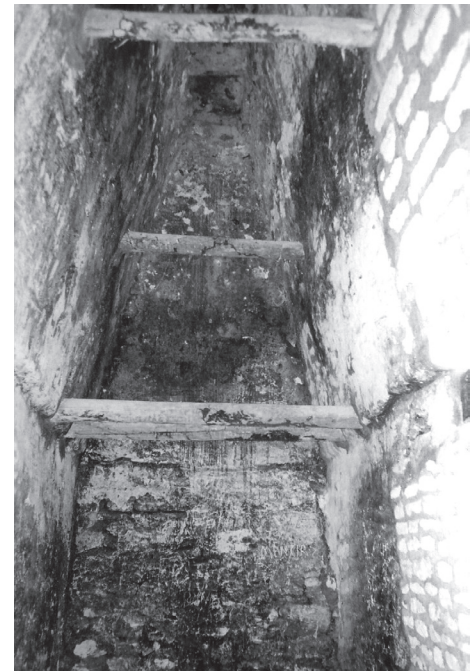
In situ Maya vault “poles” within a room with a corbelled arch, high atop “El Castillo,” at Xunantunich, Cayo District, Belize. Photo: JR.III.
