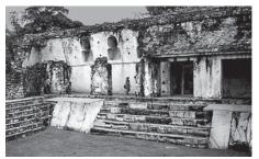
Exposed corbelled arches with groined vaults and stone lintels over doorways within the Palace structure at Palenque.
