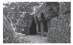
Corbelled arch and stone lintels over doorways within a structure at Yaxchilán.
