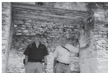
Simply-supported lintel at Caracol. Notice Jack (right) supporting the wall!
