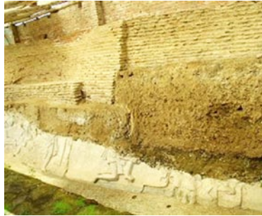
On the southeast corner of Temple 1 are exposed layers of fired-ceramic bricks and a long stucco relief made of sand and carbonized clam shells.
