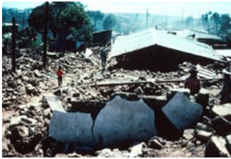
Destruction of the Patzicia district of Guatemala City by the February 4, 1976 earthquake. Collapse of the heavy adobe walls, roof tiles and beams caused most of the casualties. Slide 43, U.S. Geological Survey Open-File Report 77-165. Source: http://en.wikipedia.org
