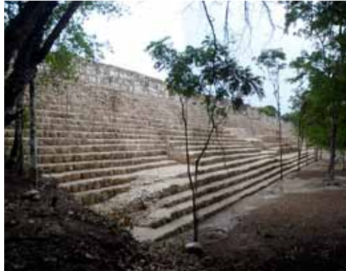
Nohochná's western side as viewed from the north. You can also see two levels of stairways, one superimposed over the other, as the structure was enlarged and enhanced over time.
