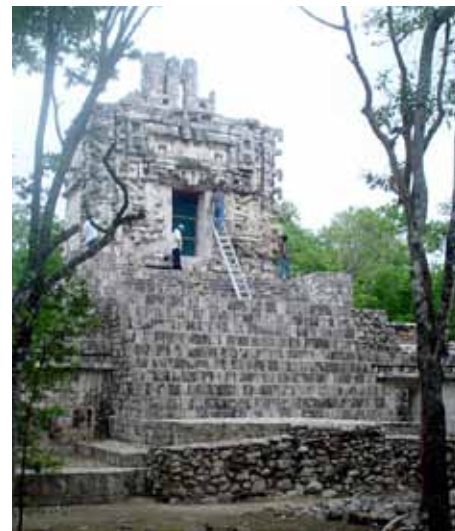
The Palace-Temple northern façade in 2009. All images courtesy of Antonio Benavides.
