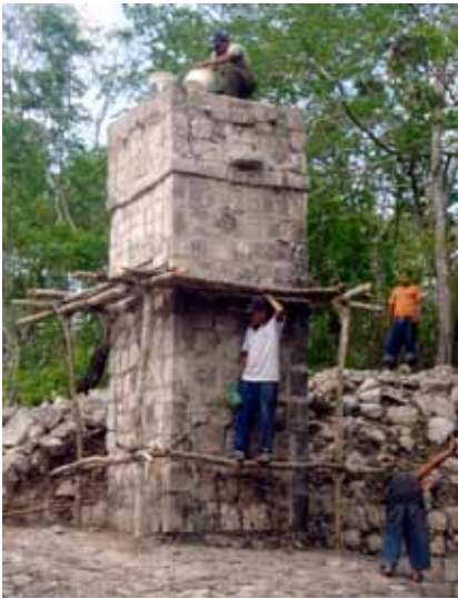
Masons working at Tabasqueño's Tower.
