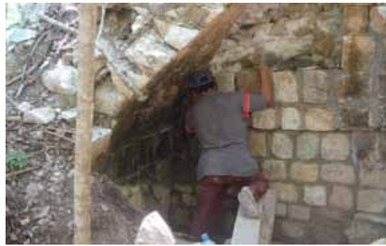
Another section of vault was consolidated to prevent its collapse.
