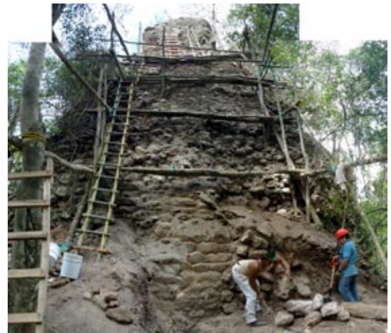
East side of Structure A2 during restoration.
