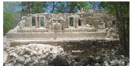
Roofcomb on same structure after restoration.
