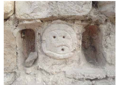
The surviving Ahau sign within roofcomb.
