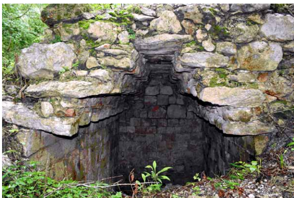
A corbeled-arch ceiling within a buried structure.
