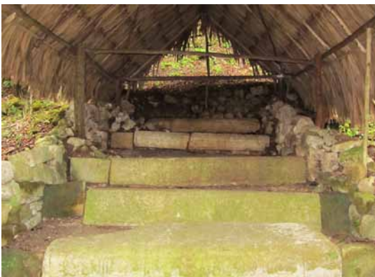
Structure L5-49 with the famous hieroglyphic steps has not been totally excavated. Today, visitors can see various step blocks protected under palapas, some of which have been replaced with replicas. Photo by Rick Slazzyk.
