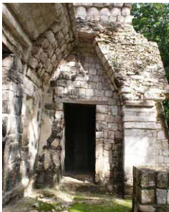
Exposed corbeled roof and wooden lintel.
