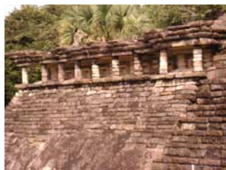
Fig. 4: Cornices and niches are almost Puuc-like in construction. All photos on this page by Joaquín J. Rodríguez, 2011.
