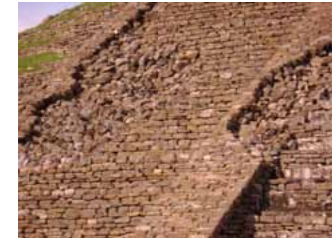
Fig. 2: River stones brought down from the mountains can be seen utilized as fill in many areas of the structure.
