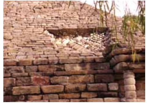
Fig. 1: The core of Structure 1 is filled with loose stones.
