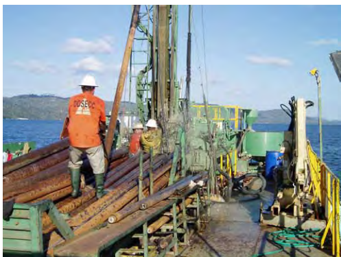
The drilling platform was working 24-hours-a-day while sediment core sampling on Lake Petén-Itzá.
