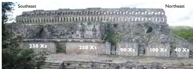
Fig. 4: East façade showing remaining panels of Xs and doorways: see Table I.
