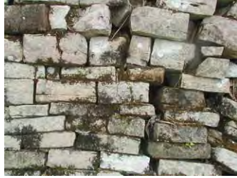
Mortarless construction (detail).
