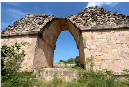
This beautifully restored corbeled arch marks one of the ceremonial entrances to the plaza at Oxkintok. Photos by Rick Slazyk.
