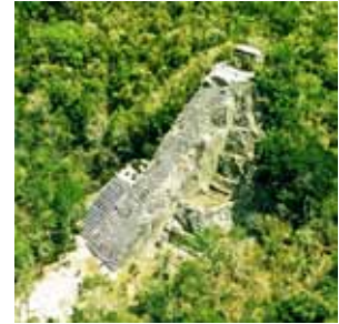
Drones are being used at Maya sites now, offering us fantastic new views. At 42 meters, "Nohoch Muul" at Coba is the tallest pyramid in the Yucatan Peninsula.
