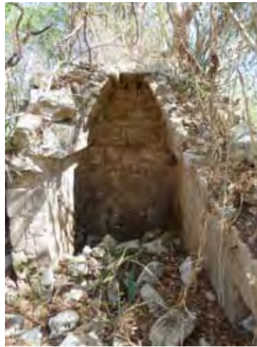
Fig. 3: Petskin, Structure I, Room 2, seen from the south.
