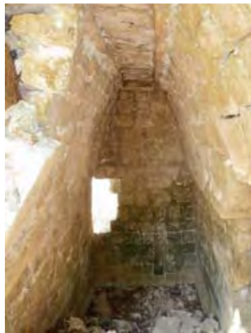
Fig. 4: Petskin, Structure I, Room I, seen from the east. All photos by Stephan Merk.
