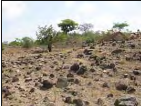
Q-40 during excavation, looking south. All images submitted by Karen Olsen Bruhns.
