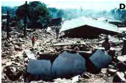
D: Patzicía destroyed. Typical street view in Patzicía, showing adobe block rubble which is all that remains of the houses that formerly lined this street. Collapse of the heavy adobe walls, roof tiles and beams caused most of the casualties. Many of the adobe blocks are still intact but the mortar between the blocks failed during the seismic shaking. Slide 43, U.S. Geological Survey Open-File Report 77-165, 1976. Public domain.
