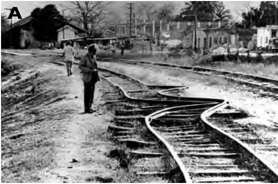
A: Bent rails in Gualán. B: Collapse of the Hotel Terminal in Guatemala City, caused by the failure of reinforced concrete columns in its third story. Both images are photos from the U.S. Department of the Interior U.S. Geological Survey professional paper 1002, published in 1976. Public domain.
