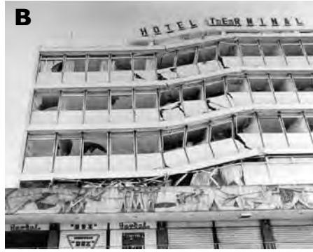
A: Bent rails in Gualán. B: Collapse of the Hotel Terminal in Guatemala City, caused by the failure of reinforced concrete columns in its third story. Both images are photos from the U.S. Department of the Interior U.S. Geological Survey professional paper 1002, published in 1976. Public domain.
