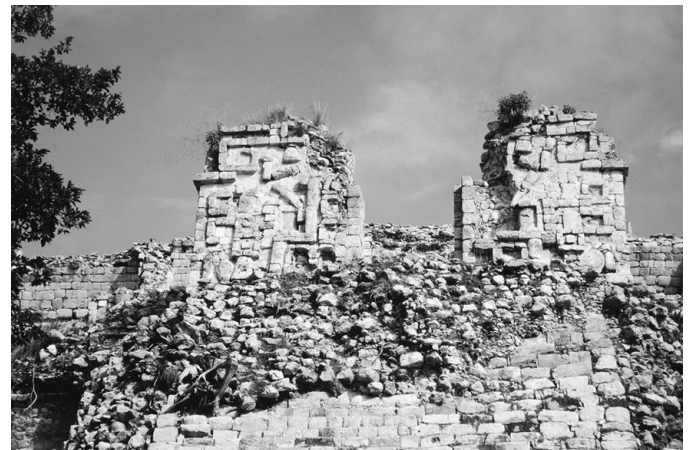
Fig. 26: The monster mouth passageway and the upper part of Stairway A are visible. (Photograph: H. Hohmann 2001)
