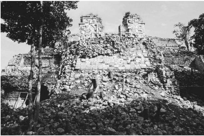
Fig. 104: The main Stairway A leads up to the monster mouth passage way. Here we can see how broad the different stairways were in relation to the breadth of the monster mouth.
