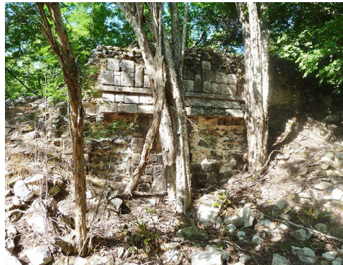
Fig. 3: Two photos of the back wall with short columns in the medial molding and single large columns embedded in the upper façade. Photos by Eduardo González Arce and Stephan Merk, 2019.
