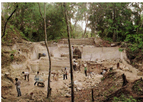
Excavation, consolidation, and restoration in the courtyard of the royal residence at Cahal Pech. Photo: Jennifer Taschek.
