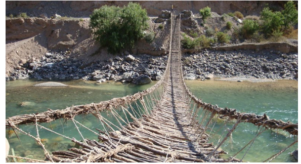
In this image, the reconstruction of the Tinkuqchaka bridge is almost complete. Photo: Cirilo Vivanco.
