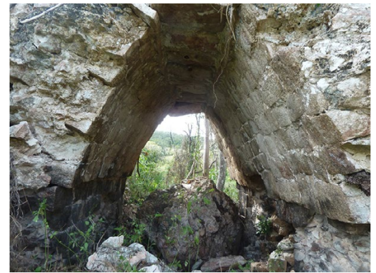
Fig. 1: A typical Classic Puuc vault in one of the northern buildings in Maler-Dsancab.
